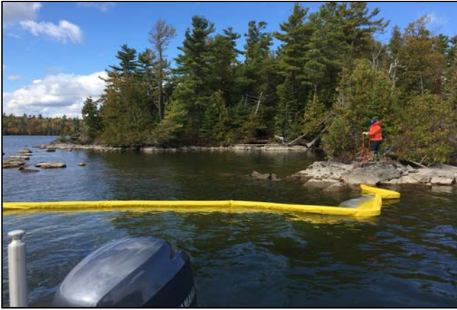
Photo 5: Placing the silt curtain at Stanley Island
