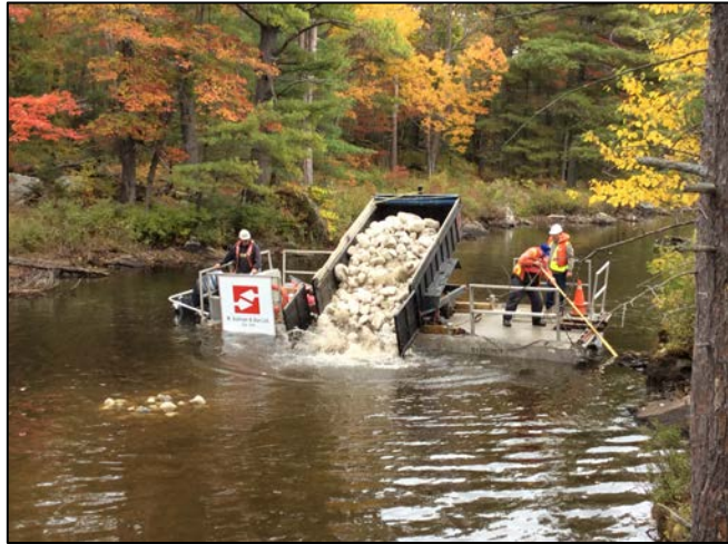
Photo 4: Unloading rock on Paris Creek Spawning Bed
